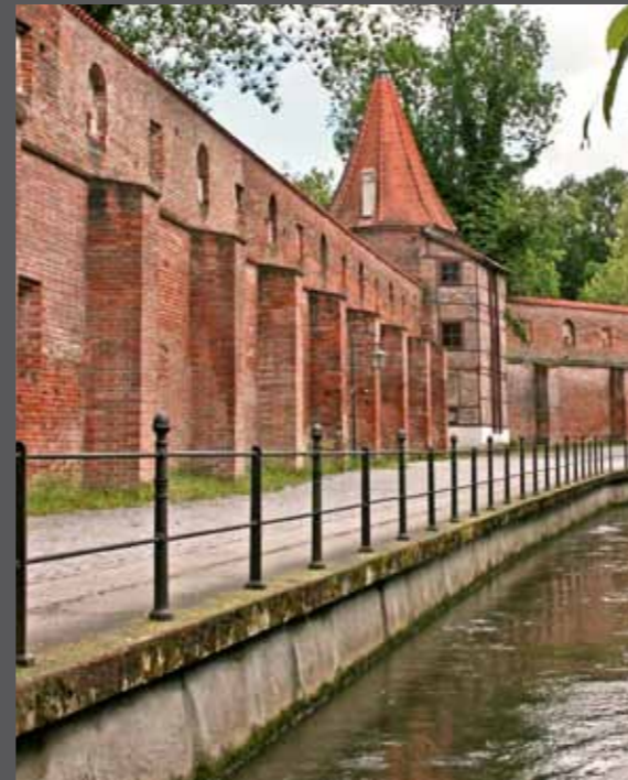
Town wall at Luginsland
