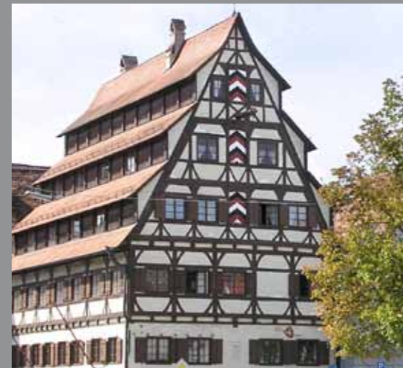
The Siebendächerhaus (House with Seven Roofs) owes its name to its unusual construction. The reason for this is that the house was used for tanning and drying skins and so they needed as many roofs as possible for laying them out. The gable is also counted as a roof alongside the six side roofs.
