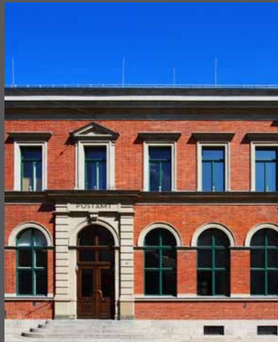
The former Bavarian Royal Post Office has been home to the MEWO Kunsthalle (art gallery) since 2005. Contemporary art exhibitions are hosted regularly here.
